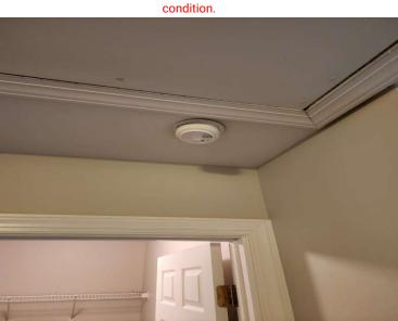
Common area hardwired combination smoke/co detector in non-compliant Common area hardwired combination smoke/co detector in non-compliant condition.
